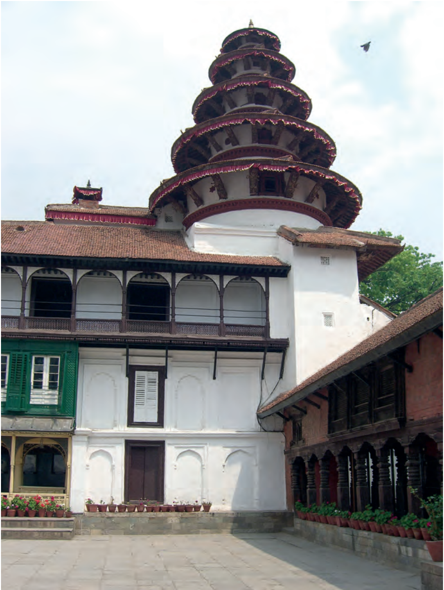
Fig. 15 The five roofs of the Pañcamukhahanumān Temple, Hanūmāṇḍhokā Royal Palace in Kathmandu. Photograph: Gudrun Bühnemann.
